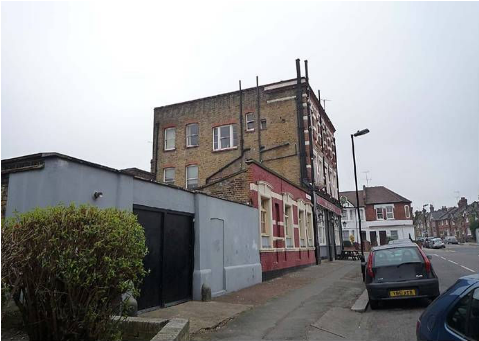
Existing Side/rear Elevation
